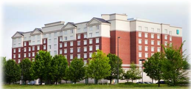
Embassy Suites Hotel in Dublin, Ohio
